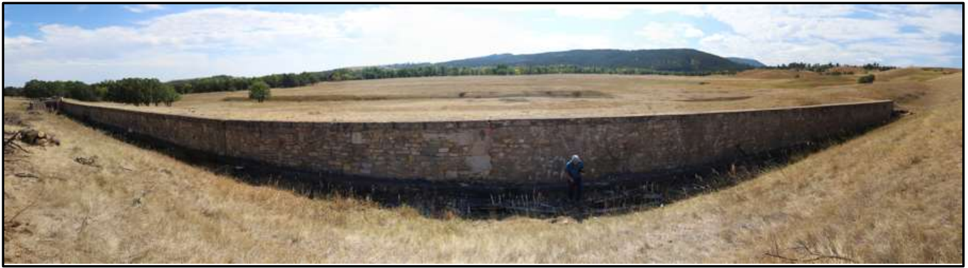
Figure 1 – Site panorama looking east (left) to west (right).
