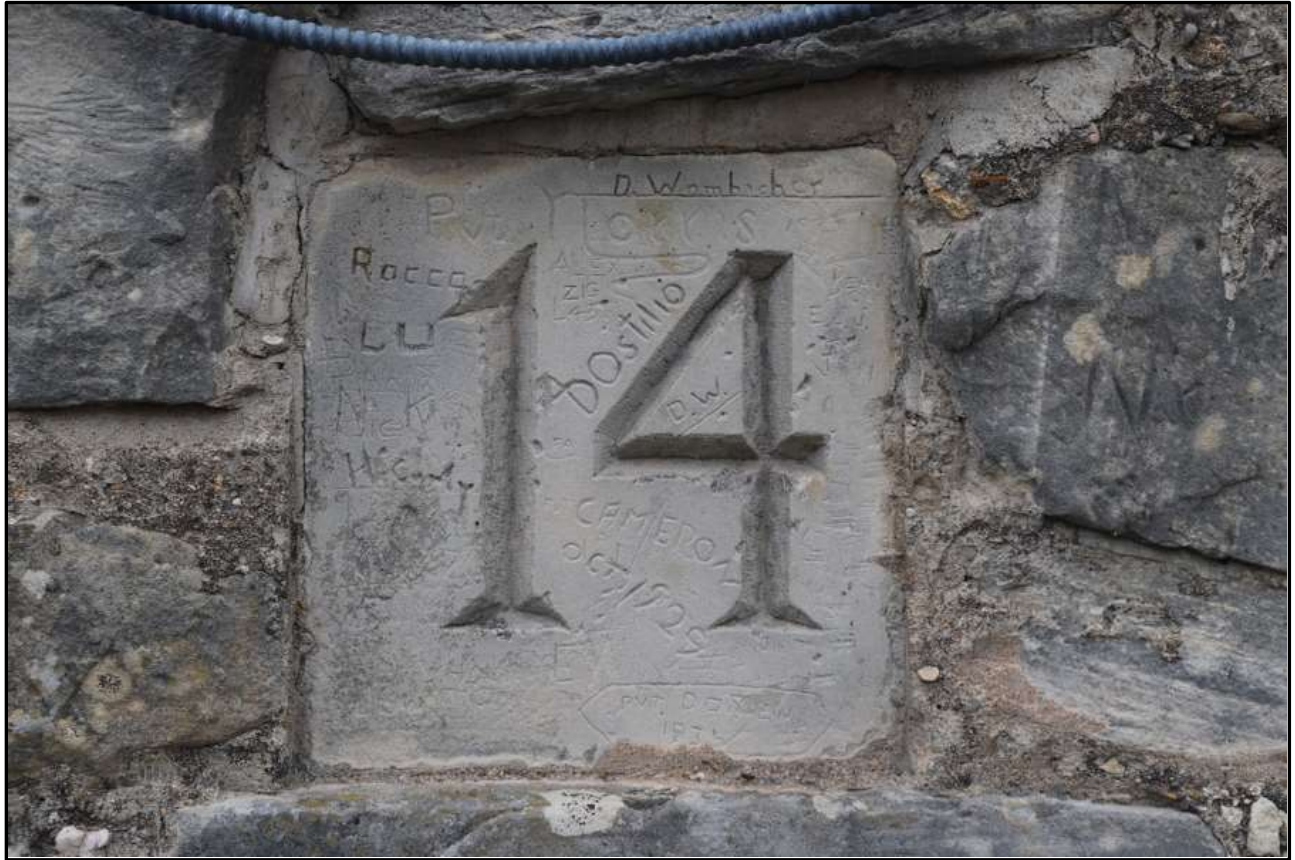
Figure 6 – The Station 14 marker incised into a sandstone block embedded in the masonry wall.
