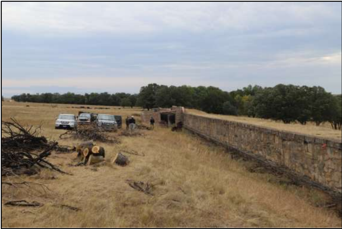
Figure 12 – Looking eastward from the west end along the back of the range wall.
